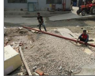
Photo of non-conformity Welding operator not using PPE.JPG
